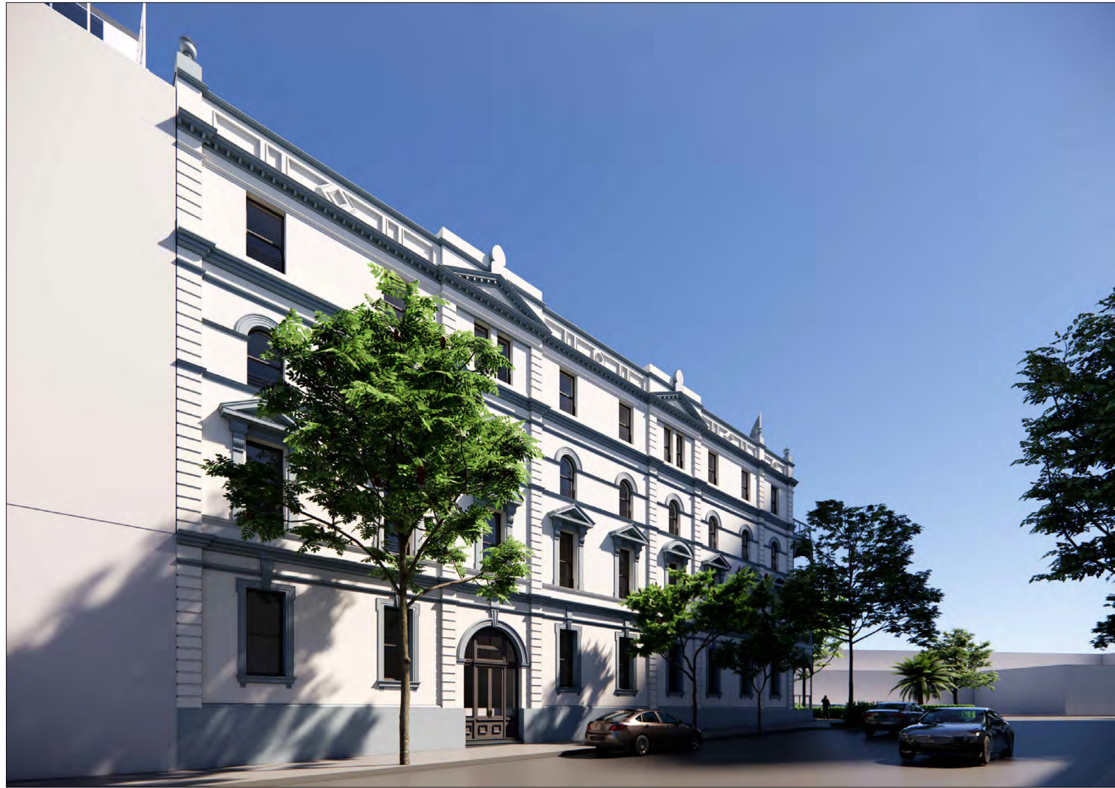
3 VIEW LOCATION F - EXISTING
