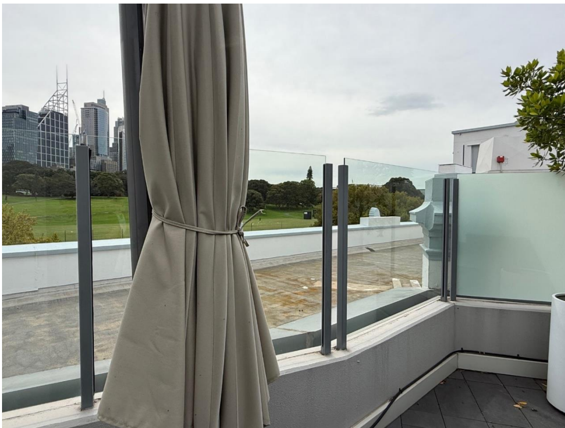
Figure 28: terrace viewed facing north/west at Unit 52/62-68 Sir John Young Crescent
