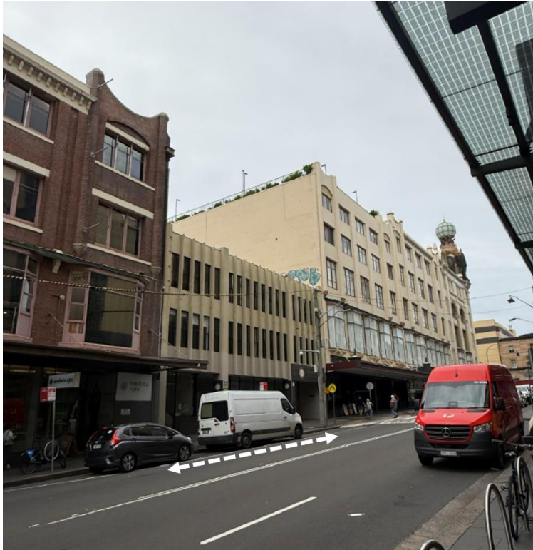
Figure 3: Site viewed from Bay Street, looking south-east
