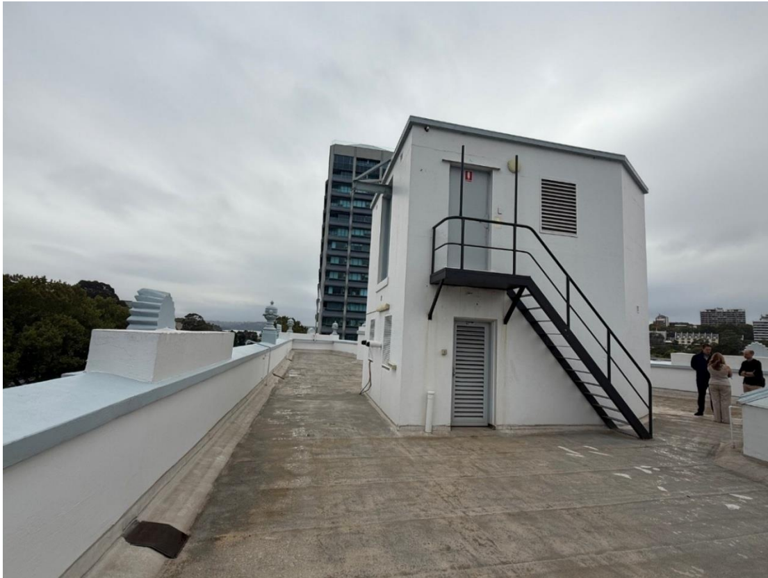
Figure 9: Existing rooftop looking north
