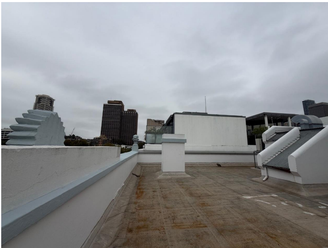
Figure 8: Existing roof top looking south-east
