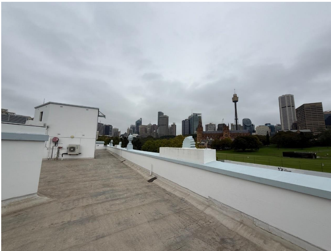
Figure 10: Existing rooftop looking south - west
