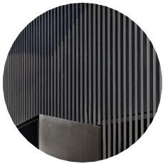
6. SERVICES METAL BATTENS ALUMINIUM PVDF FINISHED IN CHARCOAL TONE OR SIMILAR
