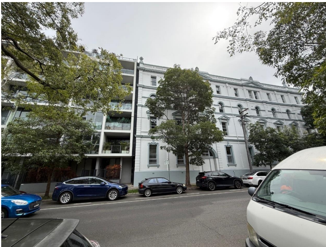
Figure 6: Site viewed from Crown Street
