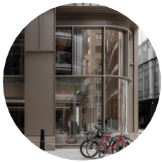
8. GF GLAZING ALUMINIUM FRAMED LOW IRON GLAZING
