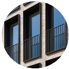
9. ABOVE GF GLAZING ALUMINIUM FRAME SYSTEM PVDF IN CHARCOAL TONE OR SIMILAR WITH HIGH PERFORMANCE IGU
