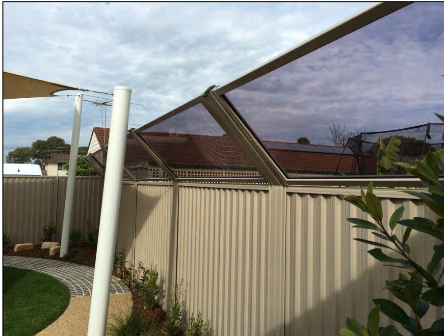
Figure 5 Example of angled barrier section
