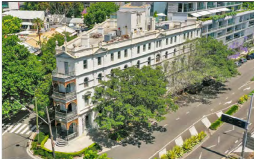
Figure 3 Subject building, including view of the rooftop the subject of this application (Source: The Palms Design and Trade)
